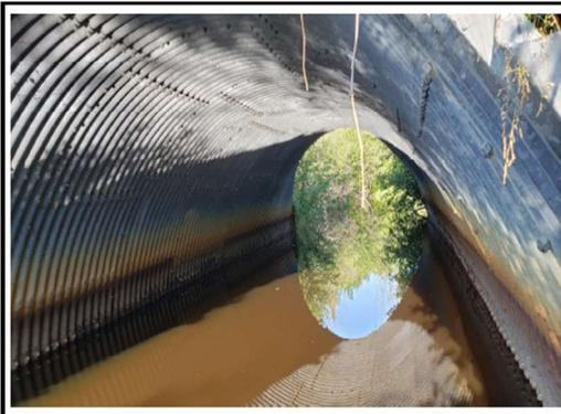
Photo 10 Moderate corrosion at waterline of barrel
