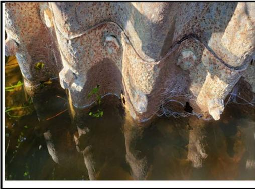
Photo 9 Perforations at the east end of culvert
